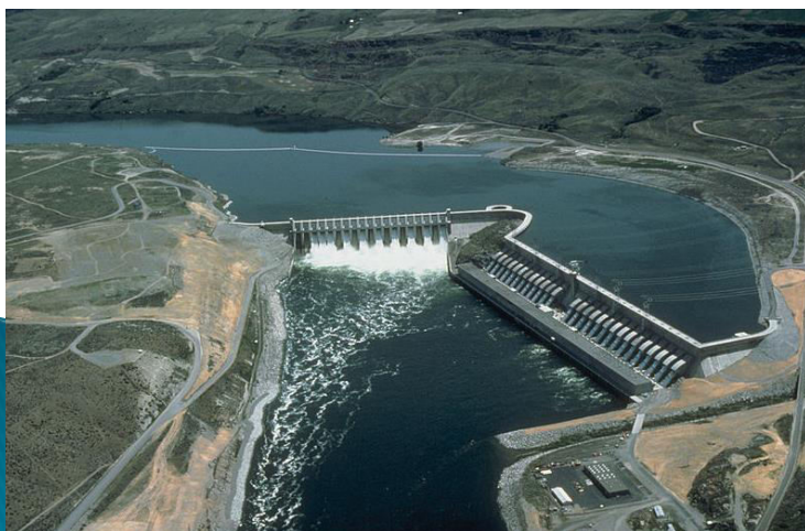
Protočna HE Chief Joseph Dam na rijeci Columbia, USA, instalirana snaga 810 MW
