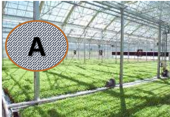
Greenhouse with zinc-coated steel structure and glass covering (Greenhouse “A”).
