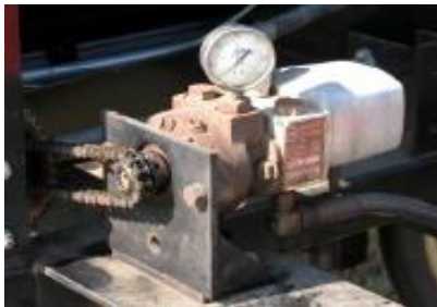
Hydraulic Valve and Motor
